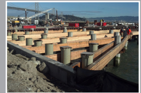
CAST IN PLACE DECKING
