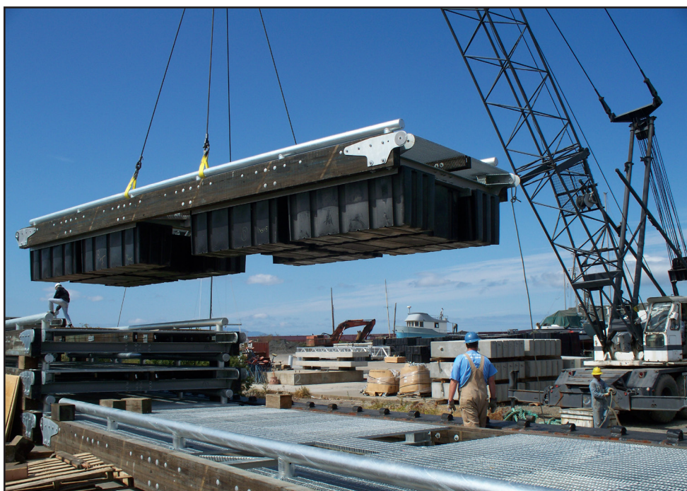
INSTALLATION OF DOCK SYSTEM
